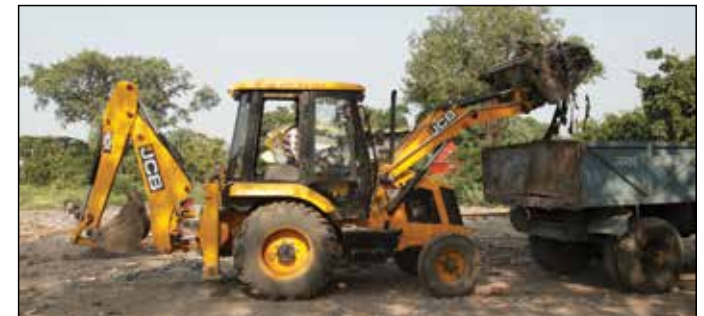
Loading with 6-in-1 bucket
