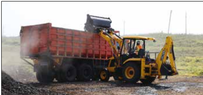
High dumper (hywa) loading
