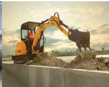
Restricted access backfilling
