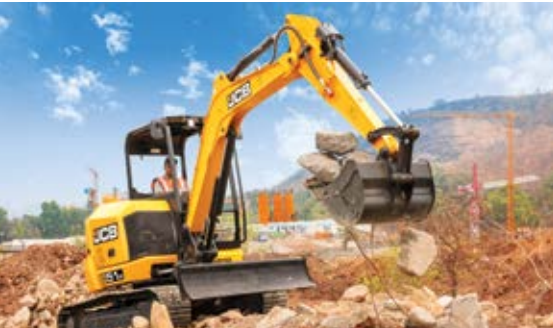
Construction site clearing
