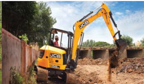
Digging close to wall
