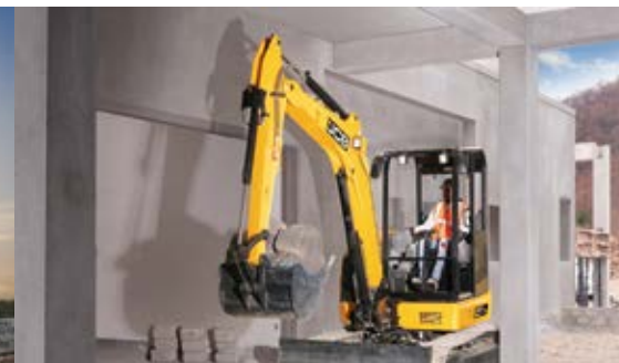
Building basement clearing
